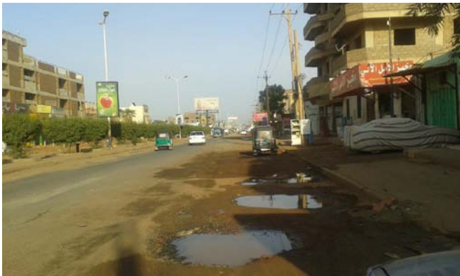
Plate 3: Ponding water on potholes
