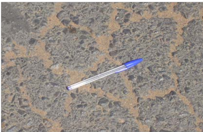
Plate 1: Alligator cracking of high severity level
