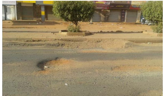
Plate 2: Severe potholes on pavement surface, [6]
