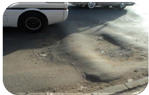
Figure 2. Severe distresses of potholes and heave
