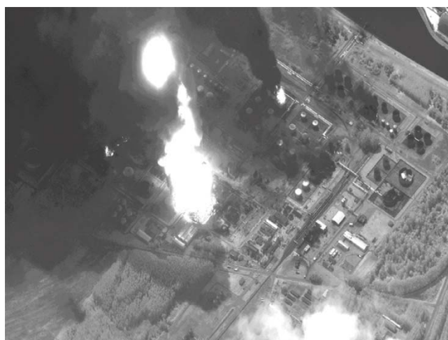
Figure 1: RNS after oil tanks were directly hit and inflamed.
